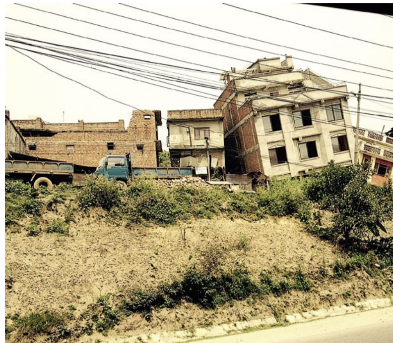
In spring 2015 an earthquake destroyed vast areas of Nepal
